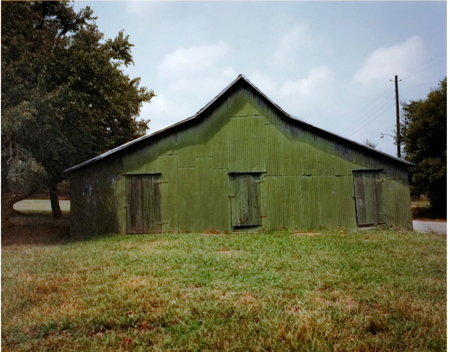
William Christenberry, Green Warehouse, Newbern, Alabama , 1978
